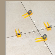
After Lavelling Process Leave Int For 8-10 Hrs.
