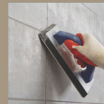
Joint Grouting
