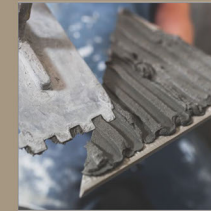
Cement Laying On Tile
