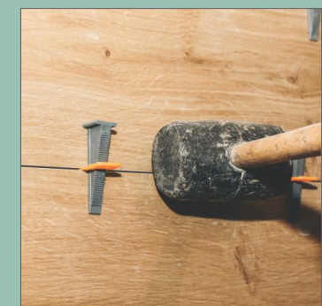
Remove Wedges Ones It Dry
