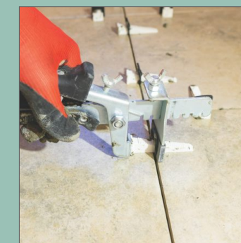
Levelling Wedges
