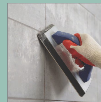
Joint Grouting
