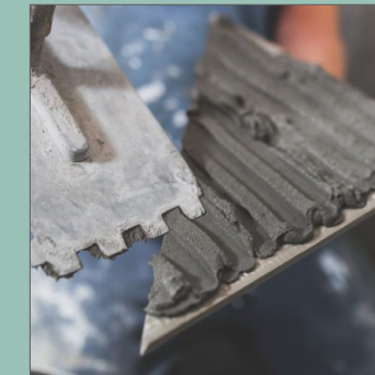
Cement Laying On Tile
