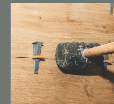
Remove Wedges Ones It Dry
