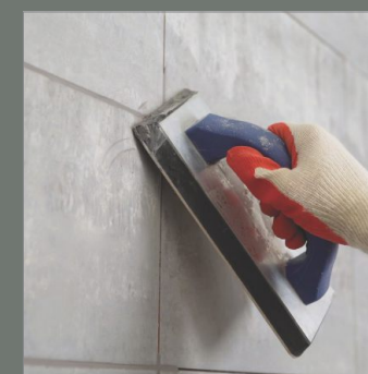
Joint Grouting
