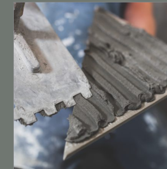
Cement Laying On Tile
