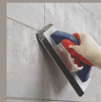
Joint Grouting
