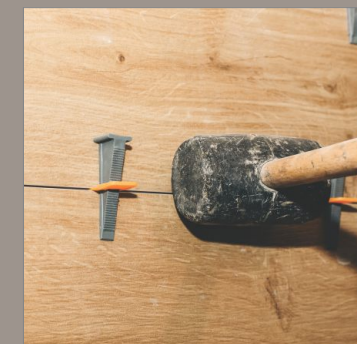
Remove Wedges Ones It Dry
