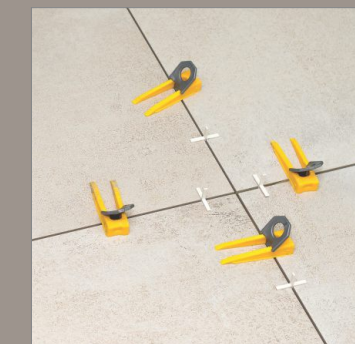
After Levelling Process Leave Int For 8-10 Hrs.
