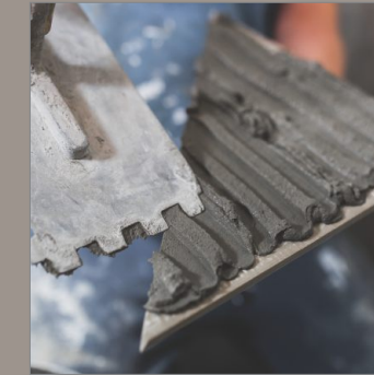
Cement Laying On Tile
