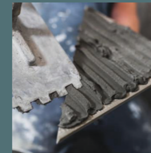
Cement Laying On Tile
