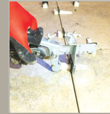
Levelling Wedges
