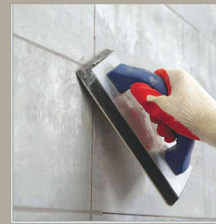
Joint Grouting
