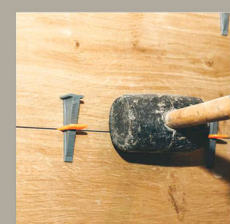
Remove Wedges Ones it Dry
