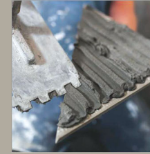
Cement Laying On Tile
