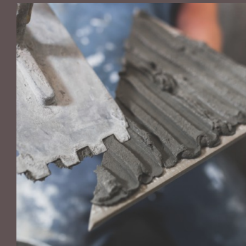
Cement Laying On Tile
