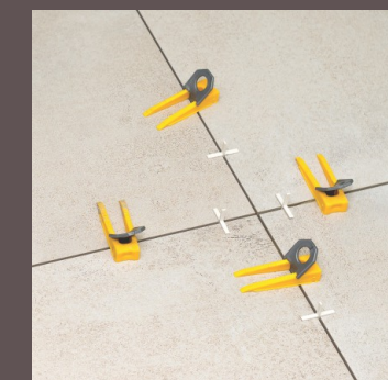
After Levelling Process Leave Int For 8-10 Hrs.
