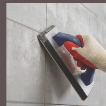
Joint Grouting
