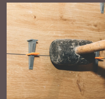
Remove Wedges Once It Dry
