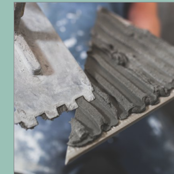
Cement Laying On Tile
