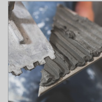
Cement Laying On Tile
