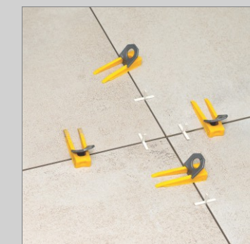
After Levelling Process Leave Int For 8-10 Hrs.
