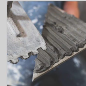
Cement Laying On Tile
