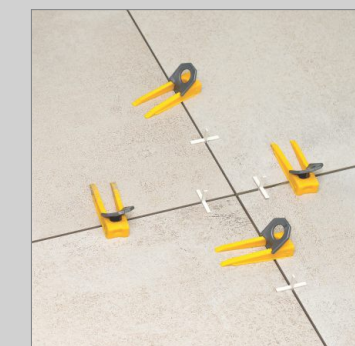
After Levelling Process Leave Int For 8-10 Hrs.
