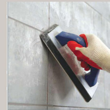
Joint Grouting
