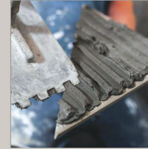
Cement Laying On Tile
